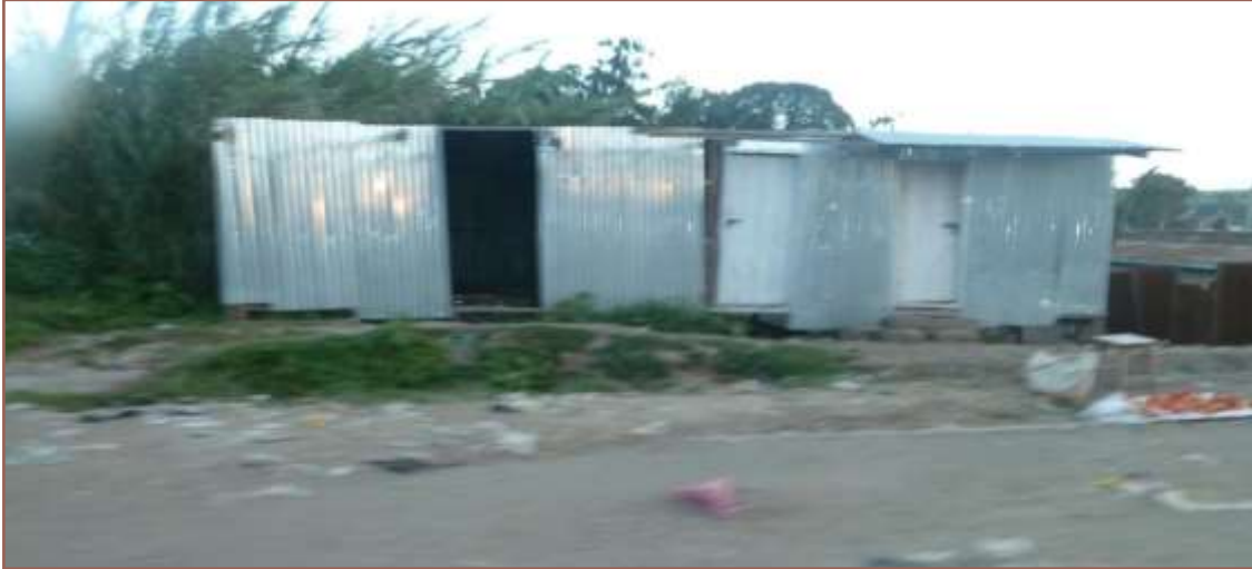
Photo 7.6: Mabati Housing Structure hanging on the valley cliff in Lower majengo
