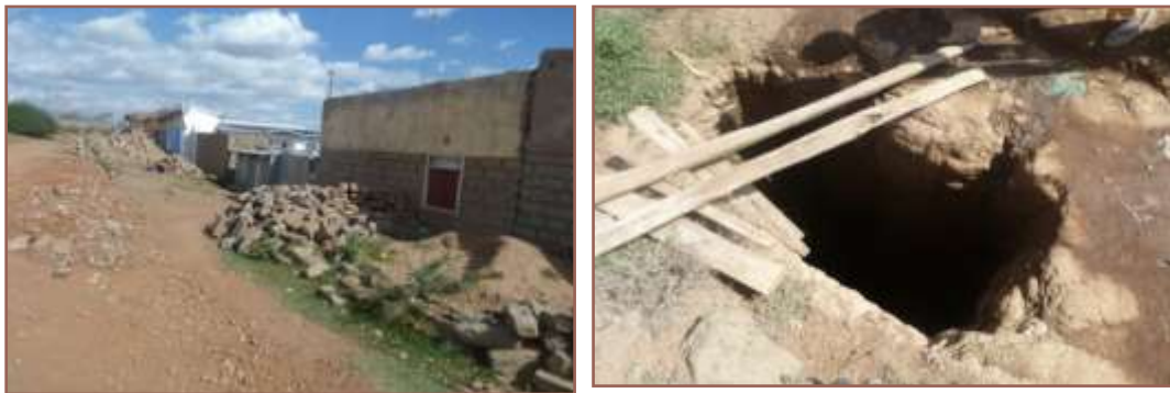
Photo 7.10: Support Infrastructure in Narok
