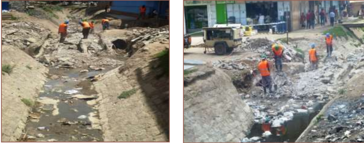
Photo 8.4: Remedial Storm Water Drainage Works on Tropical Culvert along Kakia Valley
