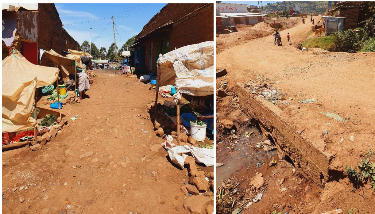
Plate 15: Poor Road Condition of Roads within the Municipality
