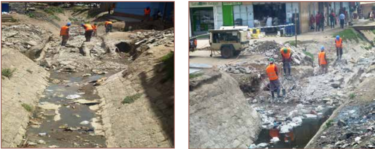
Photo 8.4: Remedial Storm Water Drainage Works on Tropical Culvert along Kakia Valley
