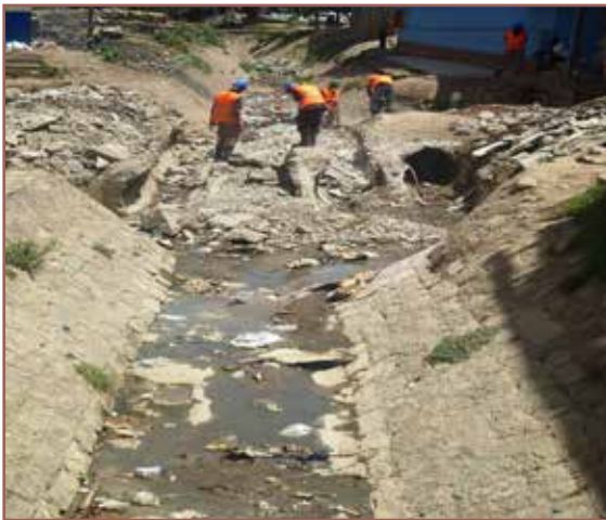
Photo 8.4: Remedial Storm Water Drainage Works on Tropical Culvert along Kakia Valley
