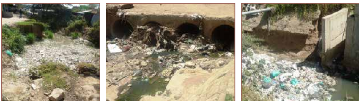
Photo 8.2: Solid waste dumped on Open Storm Water Drains
