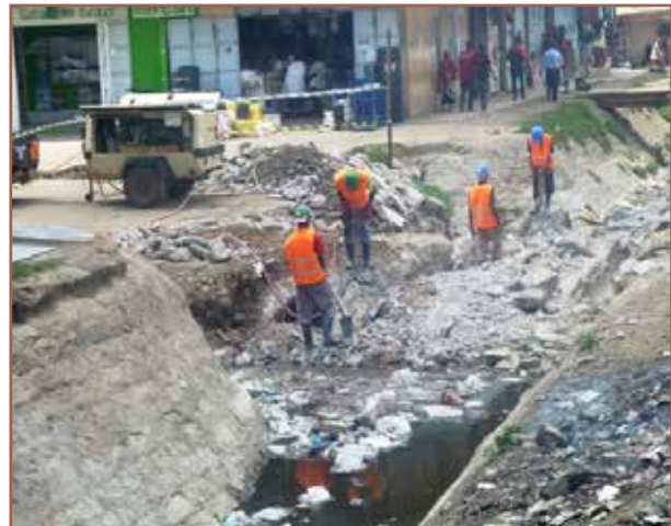
Photo 8.4: Remedial Storm Water Drainage Works on Tropical Culvert along Kakia Valley
